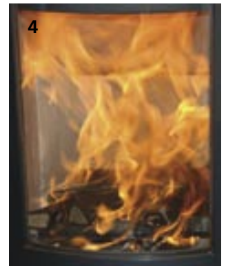
4 Large flames mean the stove and chimney will warm quickly and the fire will burn properly.
